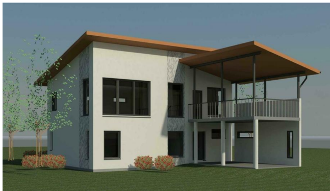
Mäntyharju zero energy building
