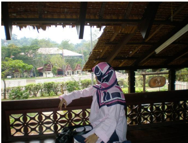
a. External balcony with a projection that provides shade and promotes natural ventilation.
