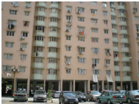
a. Vehicle-parking area
