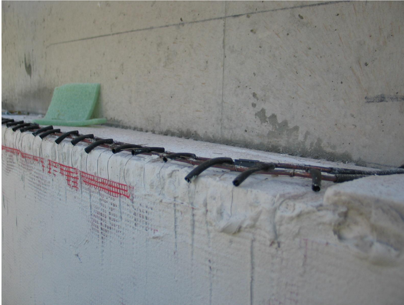
Connection of the resistance wire loops to the power supply
