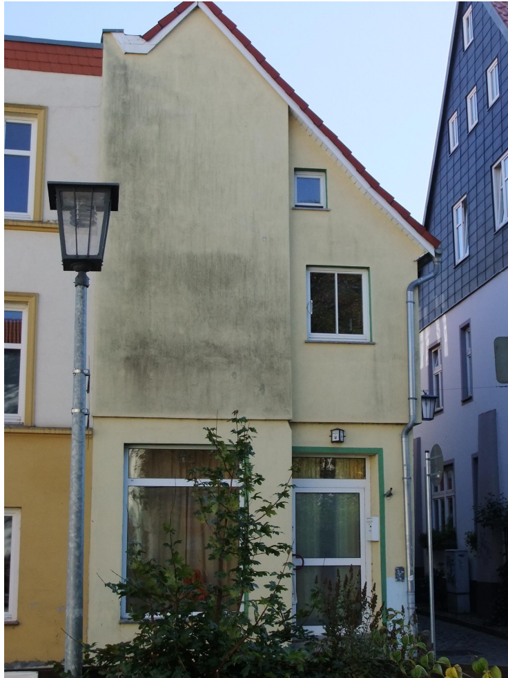
Partially insulated house in the historic city of Stralsund
