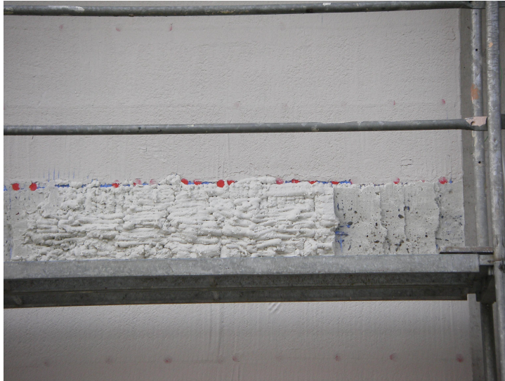
Filling of the area cut out for the piping with foam
