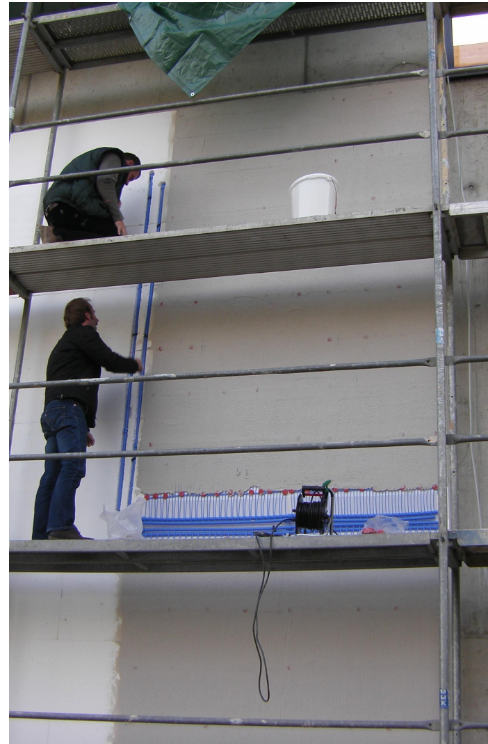
Connection of the flow and the return with the collecting pipes of the mats
