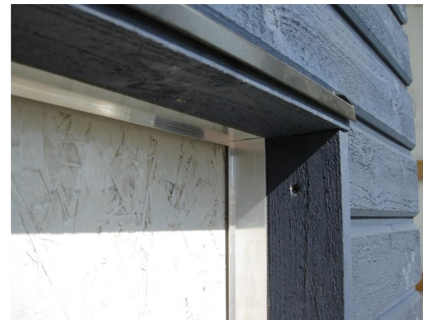
Fig. 3b. Lower right corner before covering with window sill
