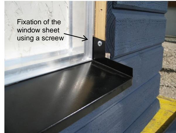
Fig. 3b. Lower right corner before covering with window sill
