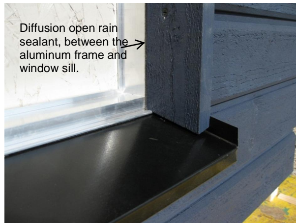
Fig. 3c. Lower right corner after mounting the window sill.
