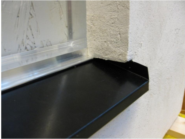
Fig. 2a. Wall with external insulation and plaster.
