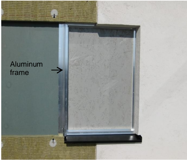
Fig. 2a. Wall with external insulation and plaster.
