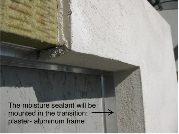
Fig. 2d. Upper right corner after plaster.
